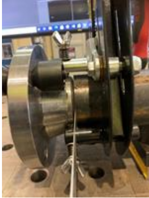
Figure 3.c: The alignment of the flange-to-pipe with metal rule inserted at junction to represent weld air gap. The wingnuts on the clamp hold the flange in place.
